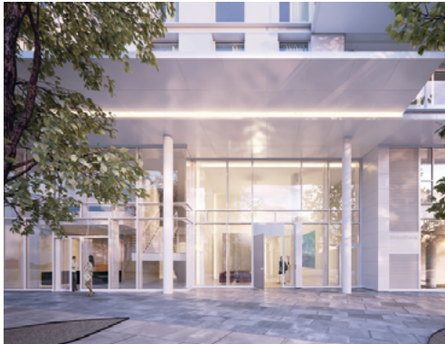
Representative entrance hall in the new building complex "Strandkai"
