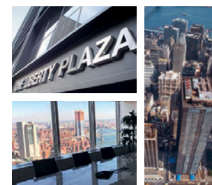
In the heart of the Big Apple Situated in Manhattan's prime location, One Liberty Plaza soars 220 metres into the New York sky.
